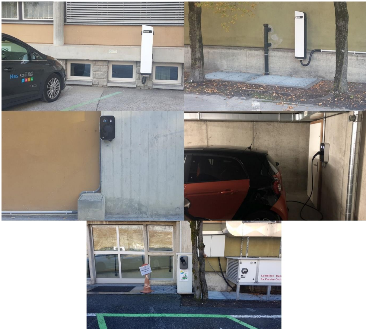
Figure 9: The two G6 (top), the two G5 (middle) and the INCH Pro (bottom) charging stations installed in Sion.
